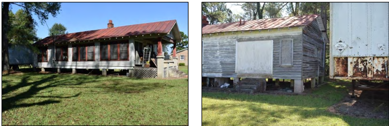
Figure 43: Left, southern elevation, right, northwestern corner (rear elevation)
