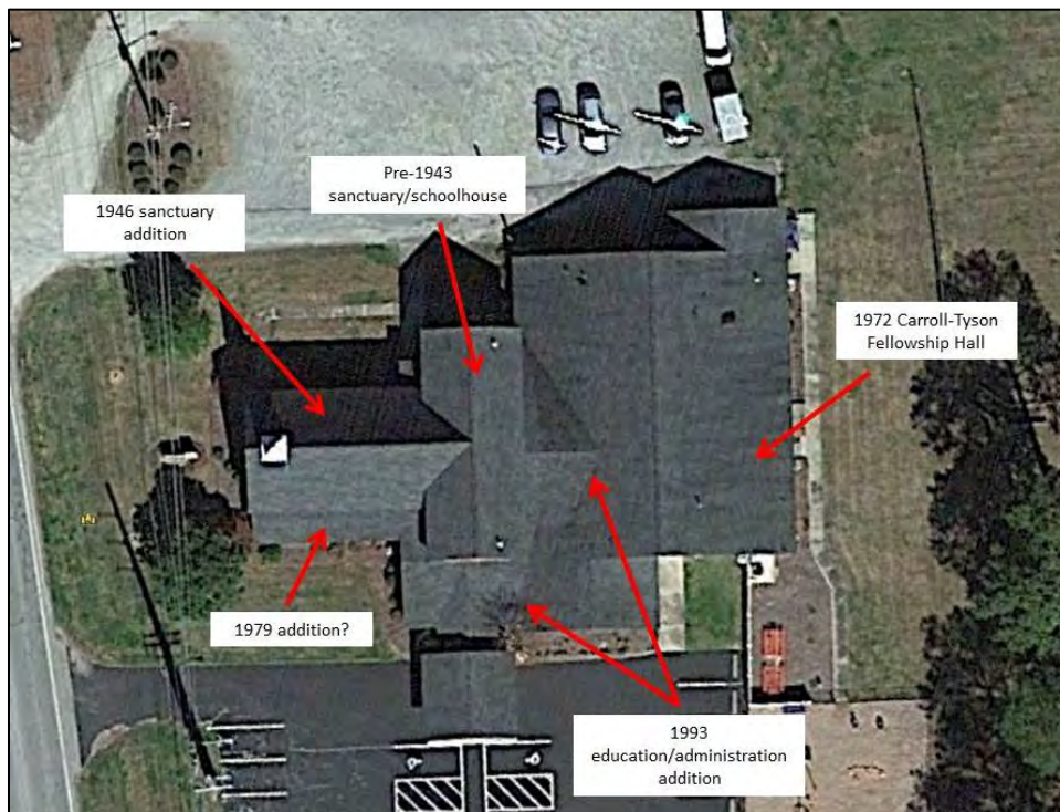
Figure 46: Modern aerial view of Hollywood Presbyterian Church
