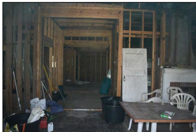
Figure 58: View of interior through front door
