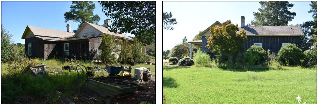
Figure 57: Left, western (rear) elevation; right, northern elevation
